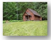
The project will encompass the completion of the roof replacement for the Suiattle Guard Station. This building is listed on the National Register or Historic Places (NRHP). Roof replacement with hand-split cedar shingles is planned to maintain the historic integrity of the building.
