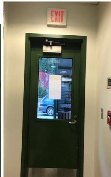
Door #1 – South Entry = Add Card Reader, REX, D/C, Electrified Strike, Change hardware to Storeroom function
