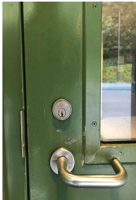
**Door #4 – East Entry = Add Card Reader, REX, D/C, Electrified Strike, Change hardware to Storeroom function**
