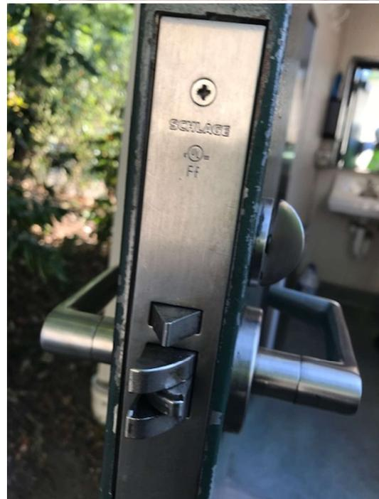
**Door 10 & 11 – Recycle = Add Card Reader, REX, D/C, Electrified Strike, Change hardware to Storeroom function**
