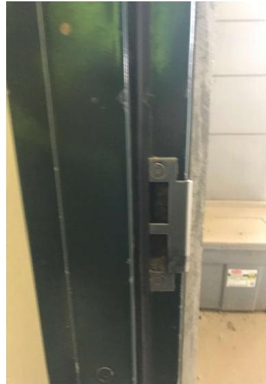
**Door #3 Vending Machine Doors = Add Card Reader, REX, D/C, Electrified Strike, Change hardware to Storeroom function. \*NOTE\*Concrete filled jam**
