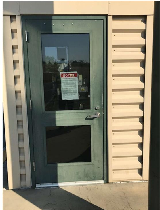
**Door 7, 8, 9 – Weight Stations = Add Card Reader, REX, D/C, Electrified Strike, Change hardware to Storeroom function**
