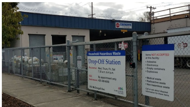
Moderate Risk Waste Facility
