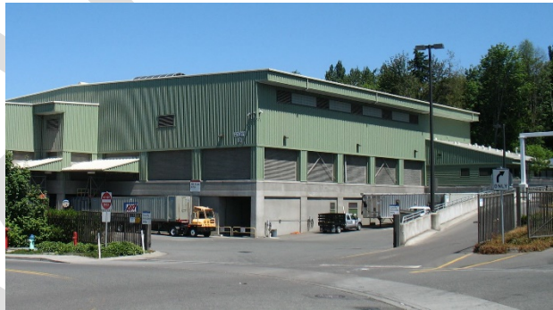
Southwest Recycling and Transfer Station
