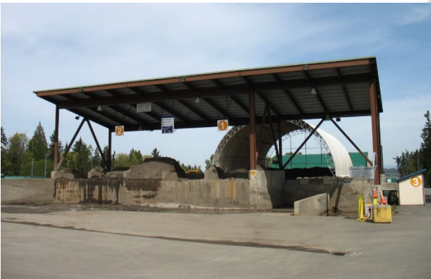
Vactor Decant Waste Facility at Cathcart
