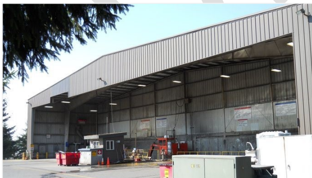
North County Recycling and Transfer Station
