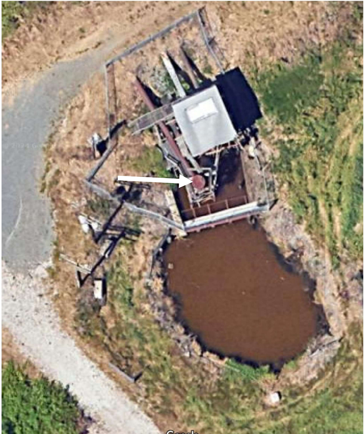
Aerial view showing submersible pump (arrow) at DD1 pump station.
