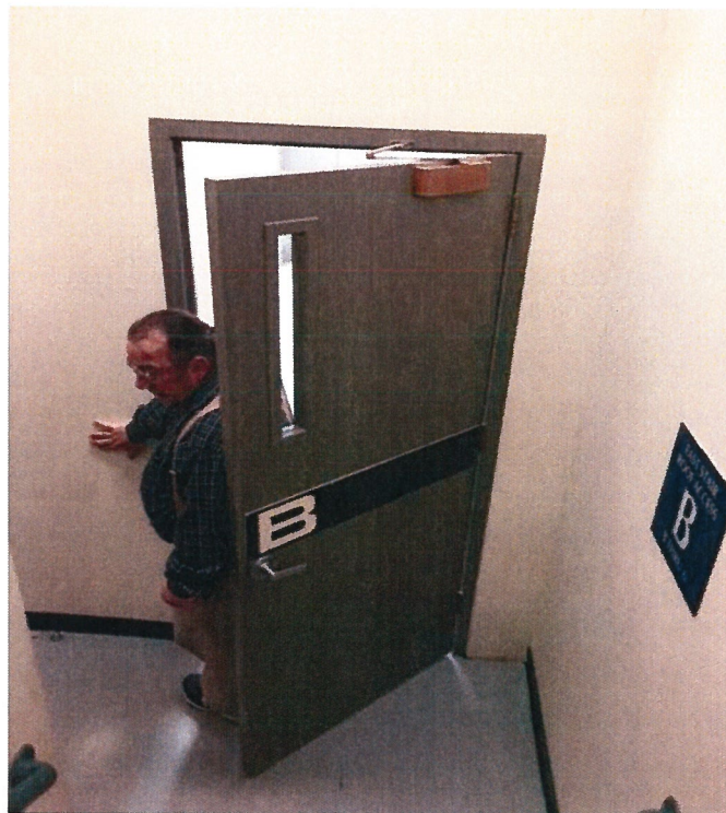
Basement Level Stairwell Door - CR location & "New" Conduit pathway
