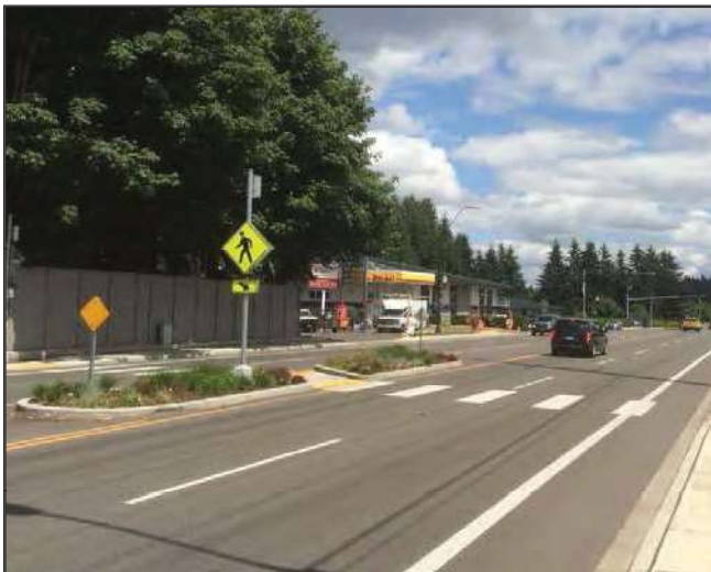
DIAGONAL MID-BLOCK CROSSING COURTESY WSDOT DESIGN MANUAL
