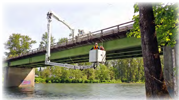
County and WSDOT inspectors in a UBIT looking at the condition of the Sultan Bridge 94 painted girders.
