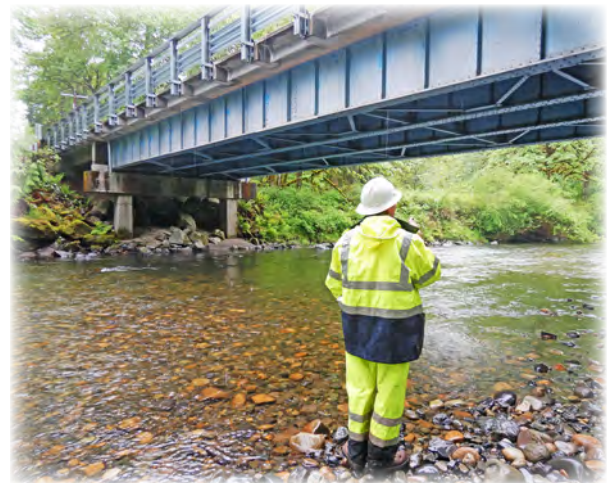
County bridge inspector evaluating the steel girders and rail system at Madden Bridge 58.
