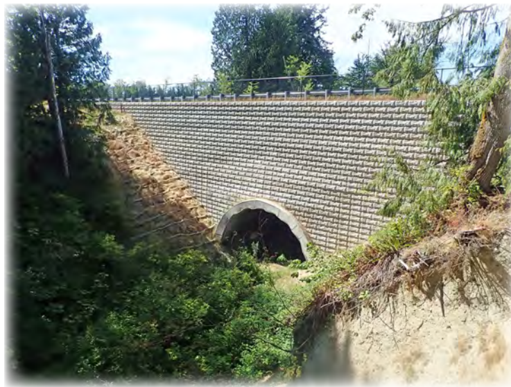
Woods Creek Vista Bridge 682 is a developer-built corrugated steel arch culvert spanning 32 feet over an unnamed creek in a new housing development just northeast of Monroe.
