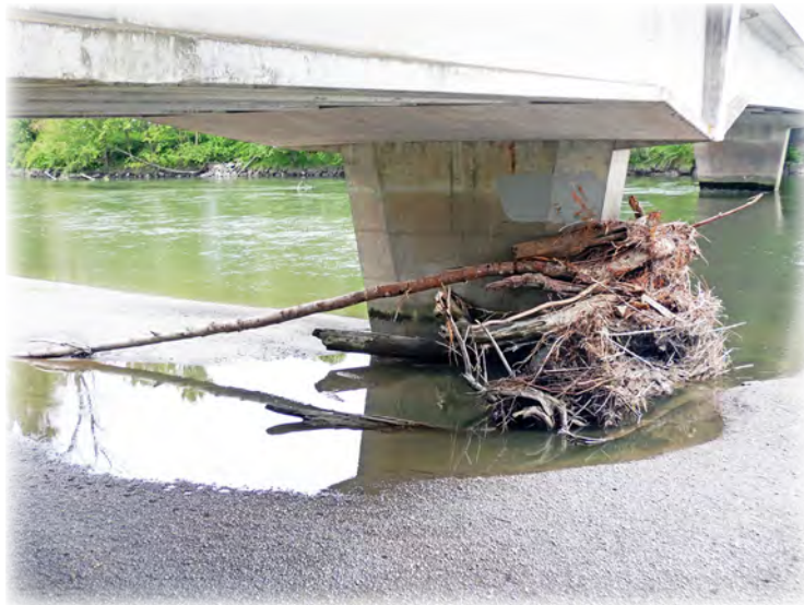
Jim Donner Bridge 4 with a log jam at one of the internal piers due to flood waters. The bridge was built over the Stillaguamish River on Marine Drive in 1985.
