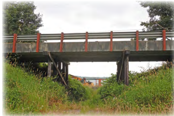
Cattle Pass Bridge 183 is a three span bridge on Lowell-Larimer Road, which was last rebuilt in 1966. The deteriorating wood substructure necessitated a load posting in 2023. The bridge is on an important agricultural and commuter route, as well as a seismic lifeline route. The county will pursue replacement funding.
