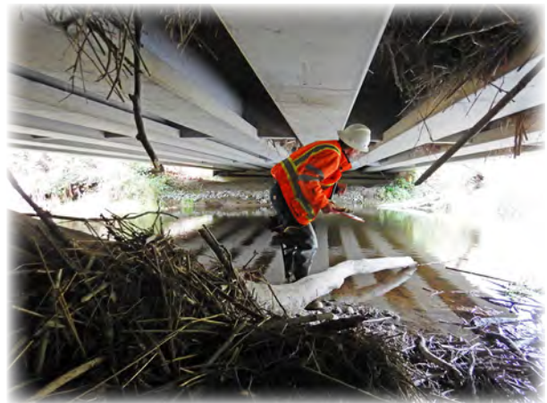
County bridge inspector under Skykomish River Slough bridge #150. High water events can cause vegetation to accumulate between the girders.
