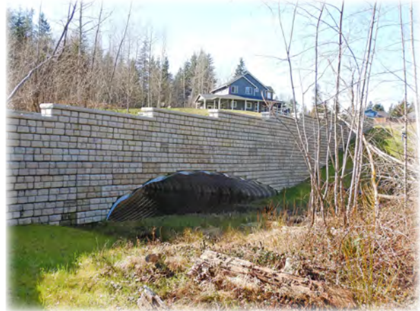
Reiner Bluff Bridge 675 is a developer-built corrugated steel arch culvert spanning 54 feet over a wetland on 120th St. SE just northwest of Sultan.
