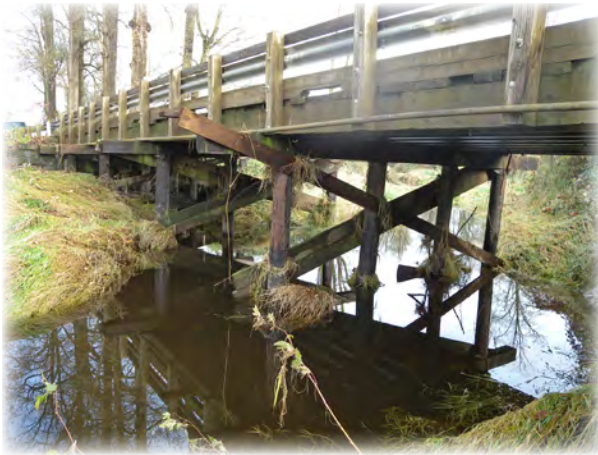
Riley Slough Bridge 52 is a four span bridge built in 1970. The bridge has a timber deck, superstructure, and substructure. Extensive repairs to the bridge necessitated a full road closure, and the condition of the substructure is poor. The county will pursue replacement funding.
