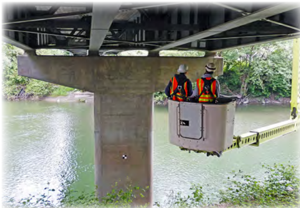
County and WSDOT Inspectors in a UBIT conducting an inspection of the steel girders at Larson Bridge 101.
