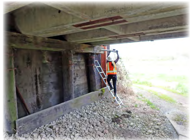
County bridge inspector drilling the timber cap at Cattle Pass bridge #190 during a routine inspection.
