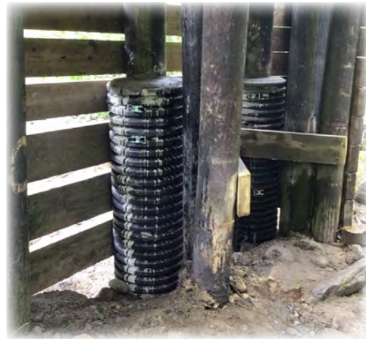
The Snohomish County Bridge Maintenance Crew is working on Silverton Bridge 56, retrofitting deteriorated piling with concrete jackets.
