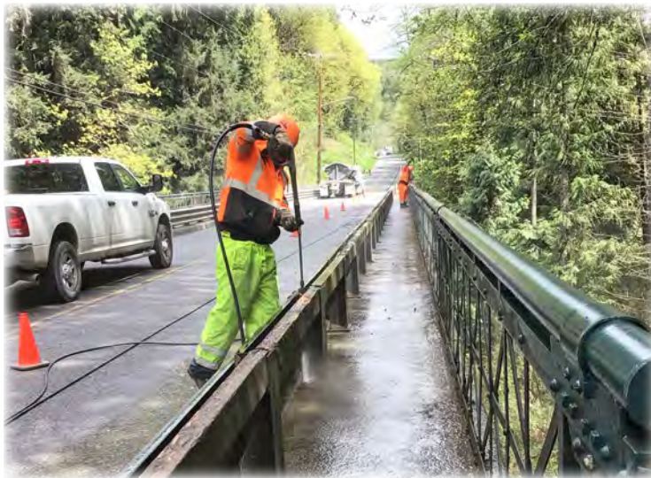
Snohomish County Bridge Maintenance Crew member pressure washing the deck and pedestrian walkway at Granite Falls Bridge 102.
