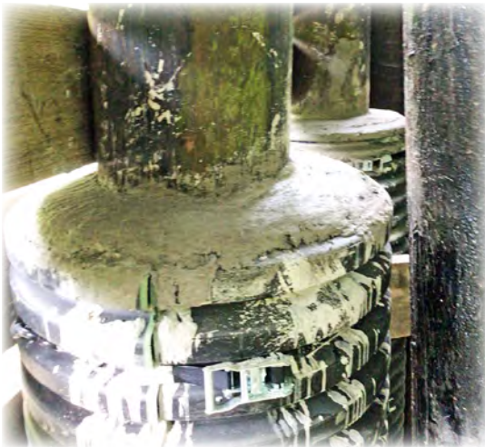
The Snohomish County Bridge Maintenance Crew is working on Silverton Bridge 56, retrofitting deteriorated piling with concrete jackets.
