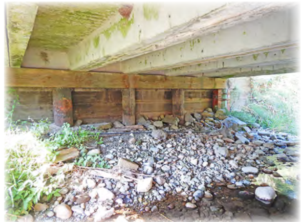
Barr Creek Bridge 158 on Ben Howard Rd located in Sultan is a short span built in 1956. It's an example of one of our bridges that is a combination of wood and concrete construction. The major rehabilitation project for Barr Creek Bridge 158 is currently in the design phase.
