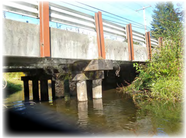
Gregory Road Bridge 272 is a two span bridge built in 1961. The bridge has a concrete tub superstructure and timber substructure. The condition of the substructure requires extensive maintenance, as it is in poor condition. The county will pursue replacement funding.
