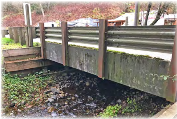
Richardson Creek Bridge 300.
