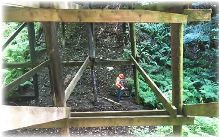
Fisher Creek Bridge 433 on English Grade Road. County bridge inspector examining timber piles and braces.
