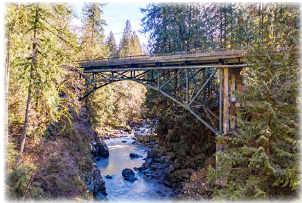
Granite Falls Bridge 102.
