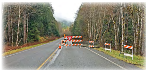
Mountain Loop Highway is currently restricted to one lane.
