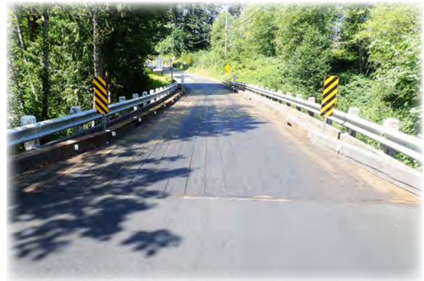
Jordan Creek Bridge 214.
