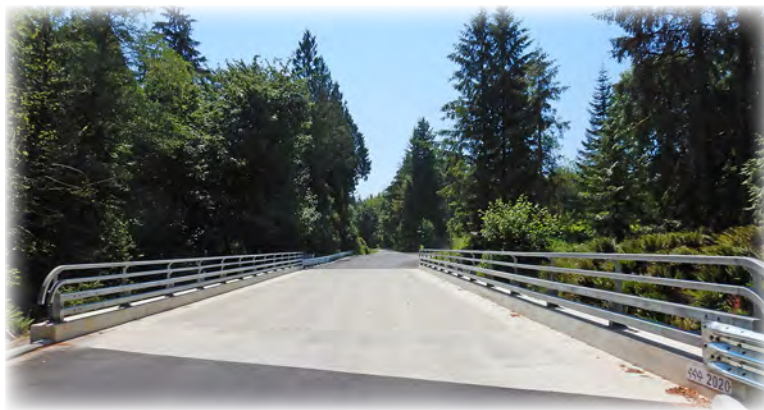
Kackman Creek Bridge No. 676 is a new 119-foot long single-span prestressed concrete girder bridge that opened in 2021. The bridge was built by the Stillaguamish Tribe in coordination with Snohomish County. The bridge carries 55th Avenue NE across Kackman Creek and replaces the old culvert, which was a fish barrier.
