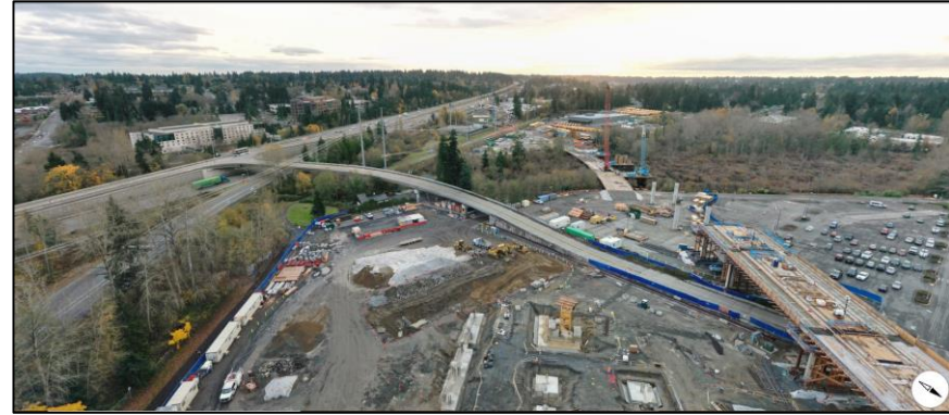
Photo: Lynnwood Transit Center Construction
