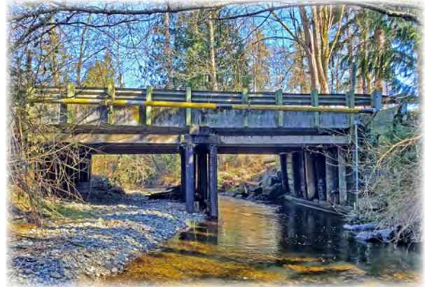
Swamp Creek Bridge 503.
