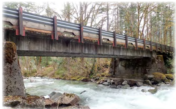
Trout Creek Bridge 494.
