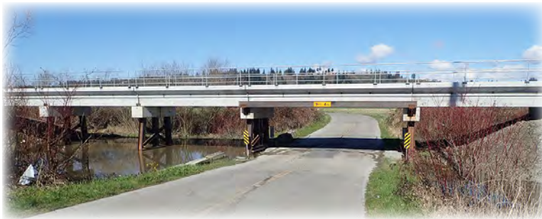
Olsen Road Railroad Underpass is height restricted. In 2019 BNSF replaced an all timber trestle with a steel and concrete bridge.
