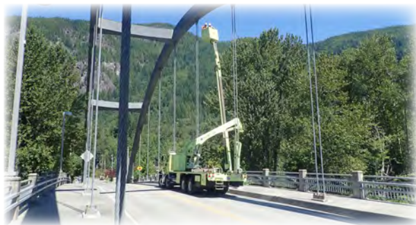
Wes Smith Bridge 122 over the N.F. Skykomish River in Index. County and WSDOT bridge inspectors inspecting the bridge’s steel arch and cables via a WSDOT UBIT.
