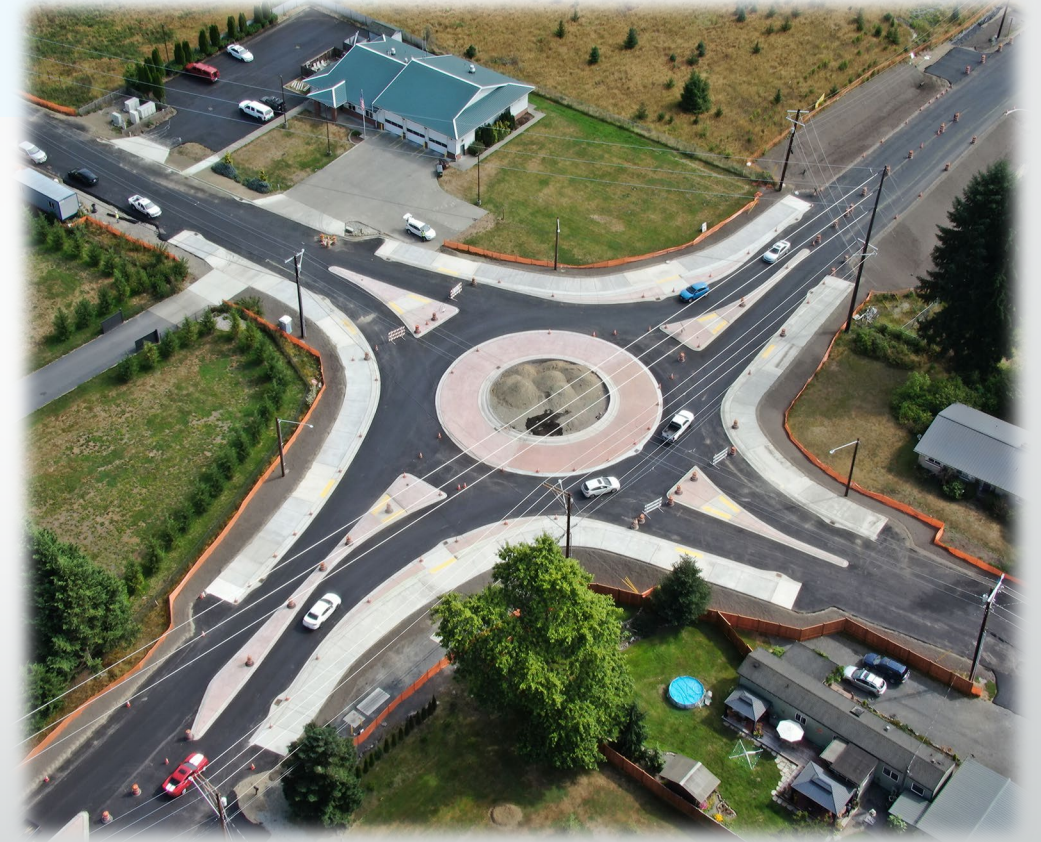
84th St NE/163rd Ave NE Roundabout
