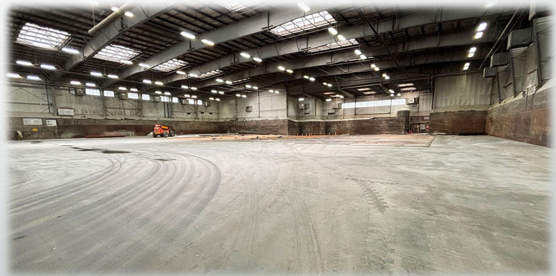
New tipping floor at SWRTS
