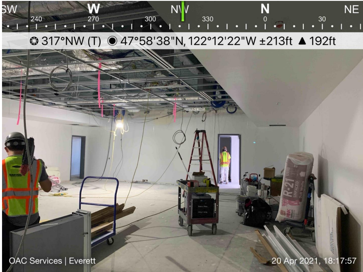
Courtroom 4A, looking north from gallery to bench, in April.
