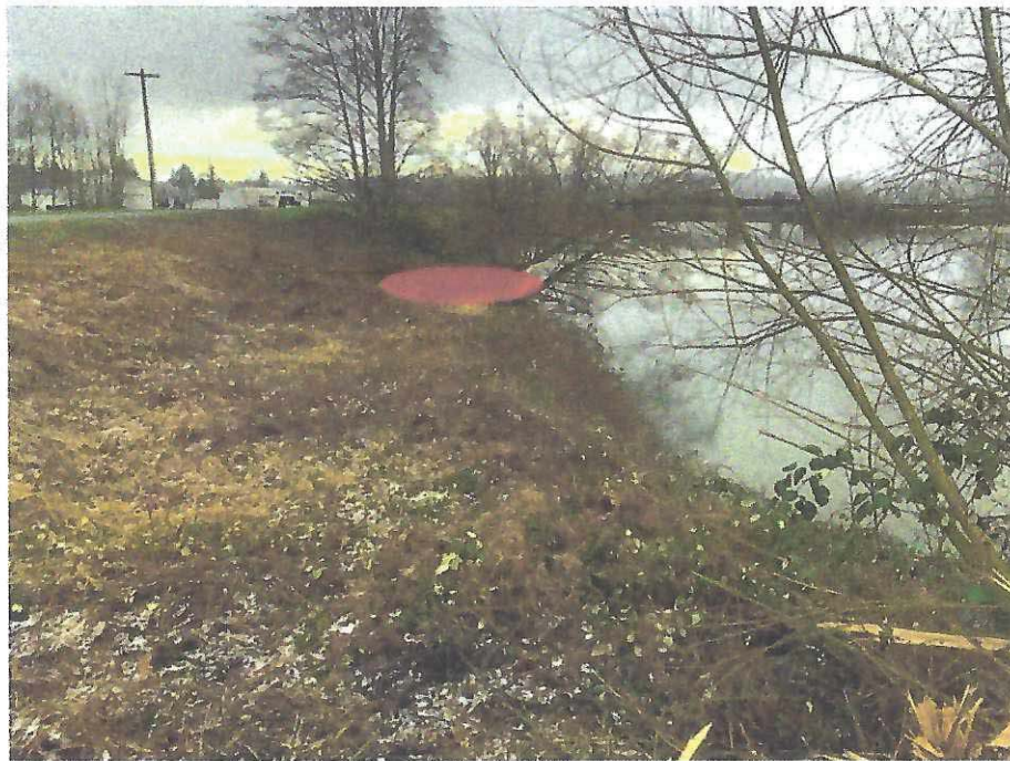
Photo D2: Scour hole, shown in red, on the riverward slope, downstream oriented (198+00).
