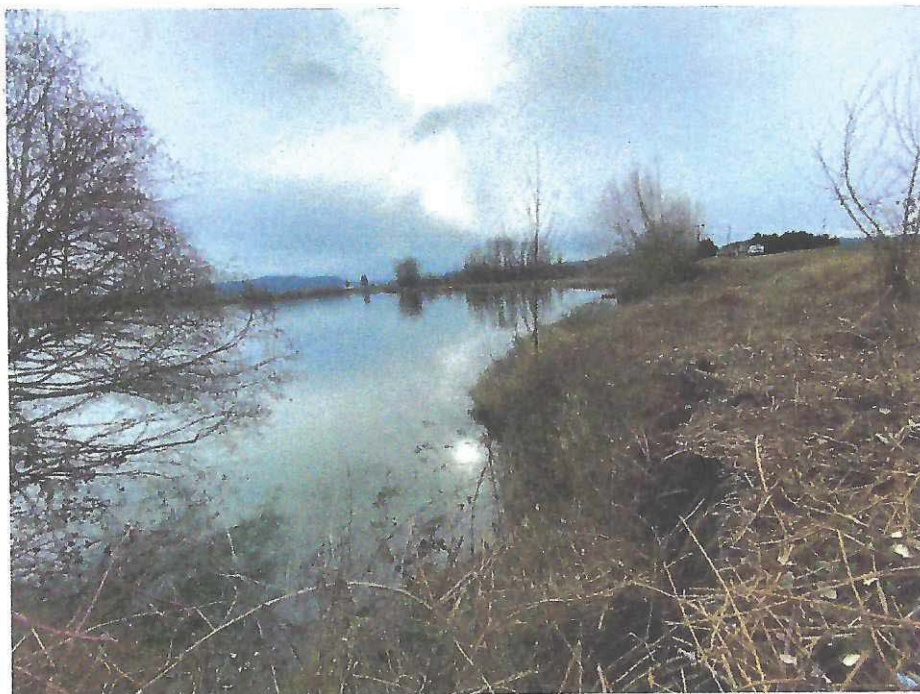
Photo D4: Scour hole and subsequent sloughing on the riverward slope, upstream oriented (STA 199+50).
