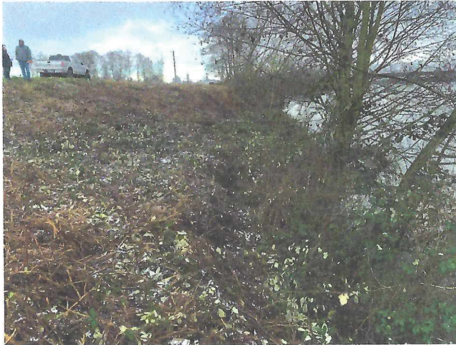
Photo D3: Sloughing landward of the trees on the riverward slope, downstream oriented (199+50).
