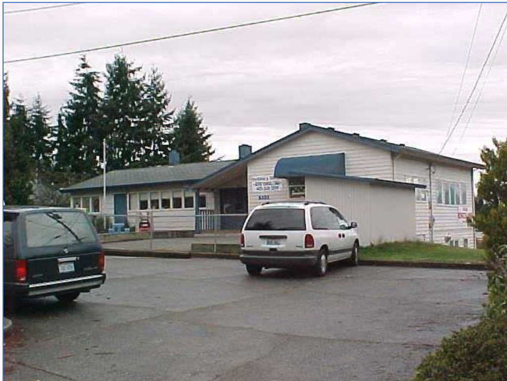
Figure 7 – Early Childhood Academy – 3,707 square feet (1,832 sq ft in basement + 1,875 sq ft on main floor)
