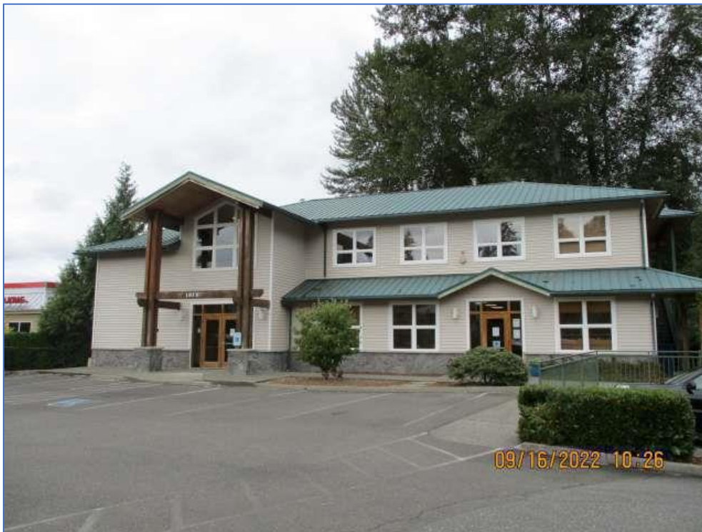
Figure 9 – Country Dawn Preschool – 5,452 square feet (2,866 sq ft on floor 1 + 2,586 sq ft on floor 2)
