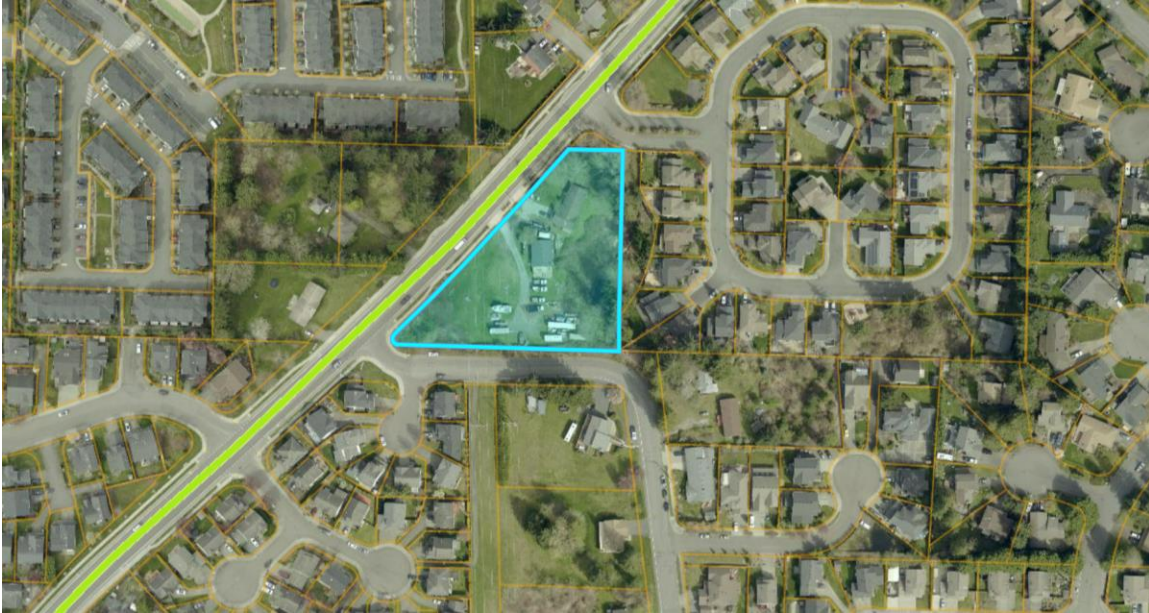
Figure 19 – Site with arterial road frontage and possible access via a local road
