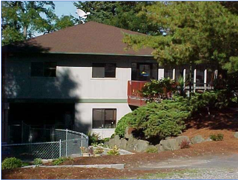
Figure 8 – Way to Grow Early Learning Center – 4,939 square feet (2,299 sq ft in basement + 2,640 sq ft in main floor)
