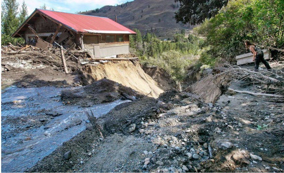
Figure 15 – A debris flow damages a structure and property in 2014 after the Carlton Complex Fires,
