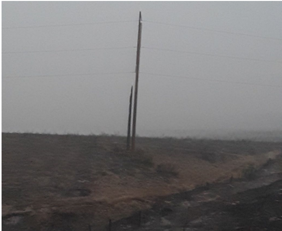
Figure 12 – Transmission lines burned by the Cold Creek Fire in Okanogan County in 2020
