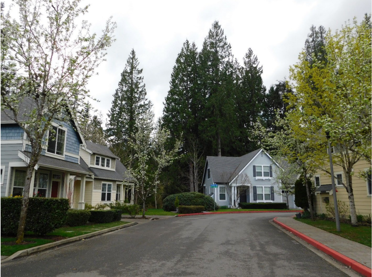
Photo 2: North Creek Condominiums, Bothell. Photo Credit PDS Staff
