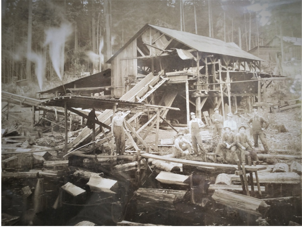
Cutthroat Creek dammed to facilitate the logging operations of the early 1900's
