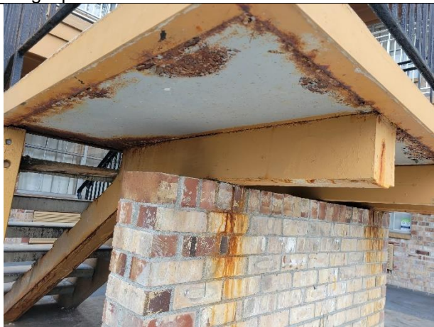
Corroded steel support for stairs
