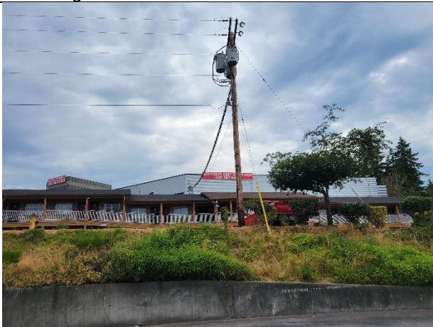
3 phase power – overhead lines
