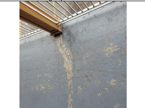
2 nd level concrete crack – trip hazard
