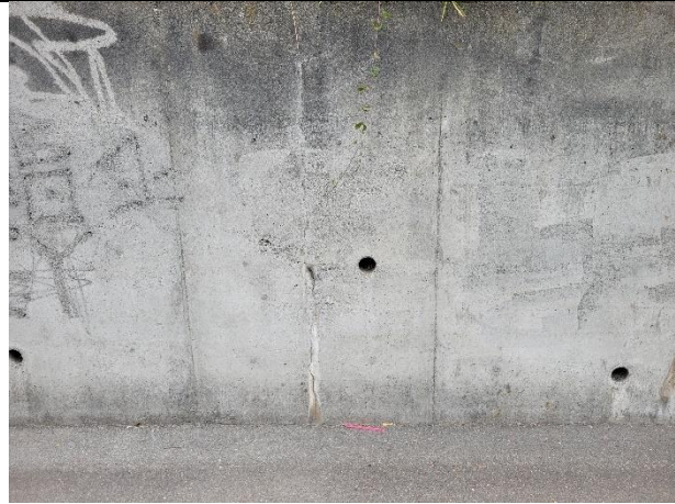
Retaining wall – some cracking
