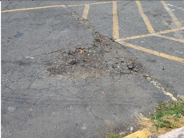
Pavement alligator cracking
