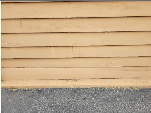
B2 siding – peeling paint and cracked siding
