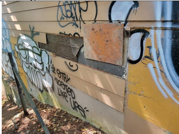
Damaged siding east elevation
