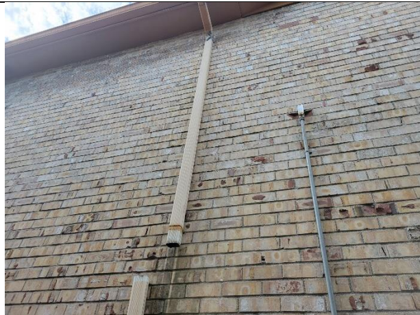
Disconnected downspout
