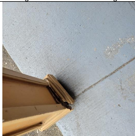
Rotted wood – column wrapping, typical
