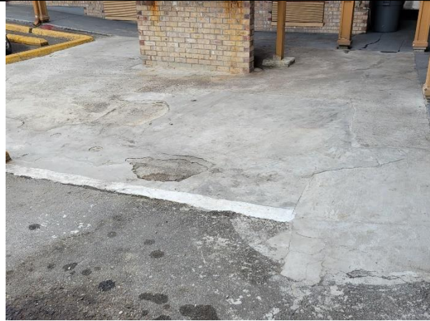
Parking area – concrete cracking
