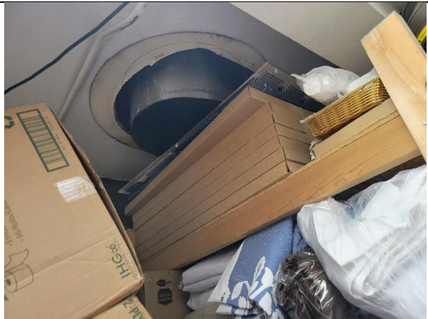
Abandoned ducting in storage area
