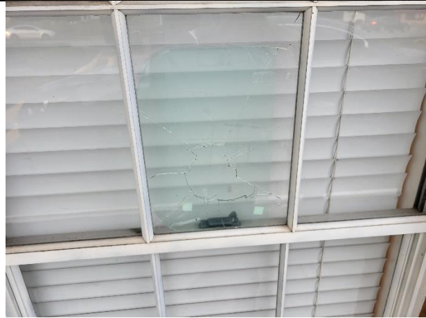
Broken window – west elevation
