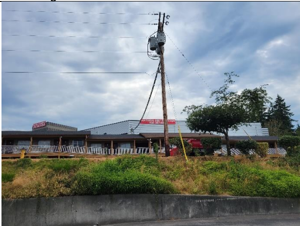
3 phase power – overhead lines
