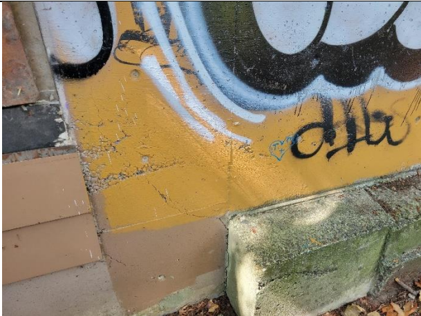
Some stem wall cracking – east elevation
