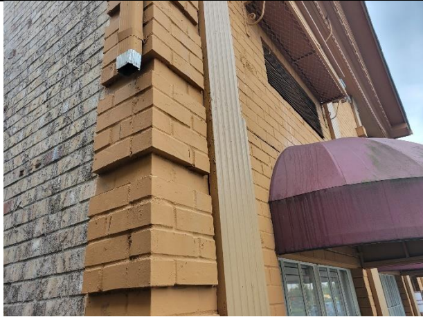
Disconnected downspout – NW corner
