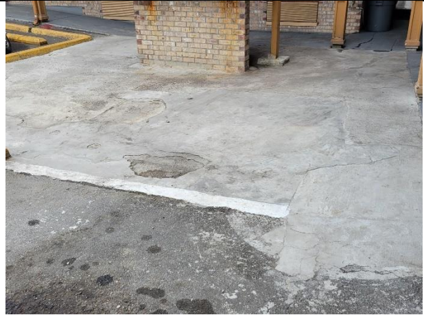
Parking area – concrete cracking
