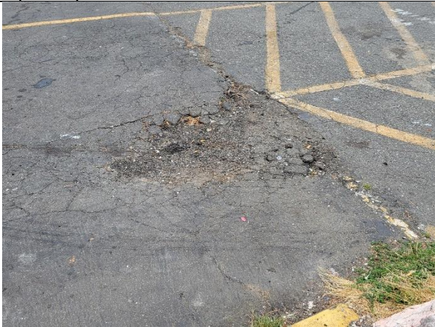
Pavement alligator cracking
