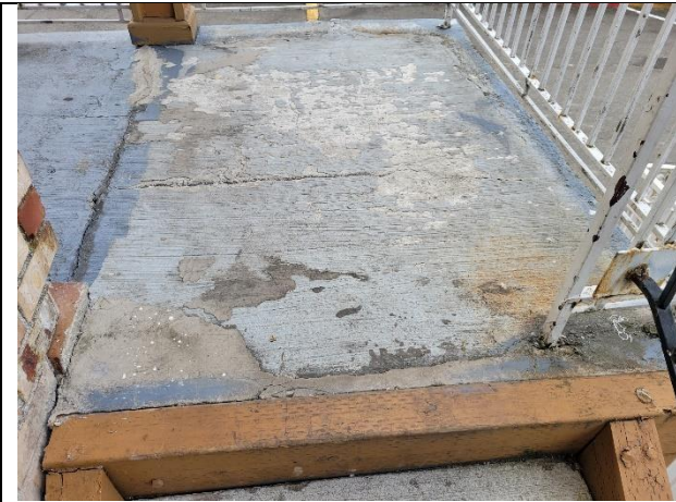
B1 2 nd floor landing – cracking concrete
