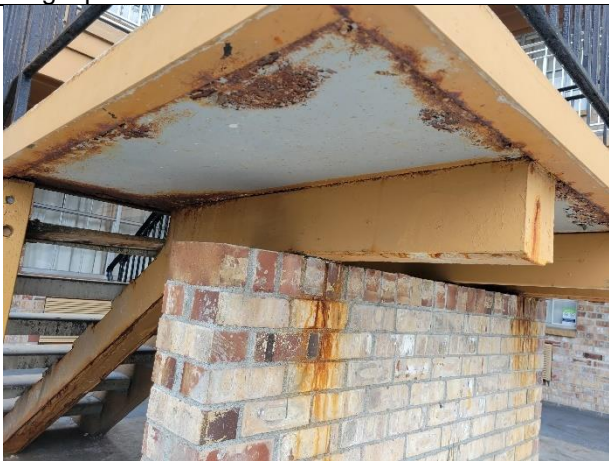
Corroded steel support for stairs
