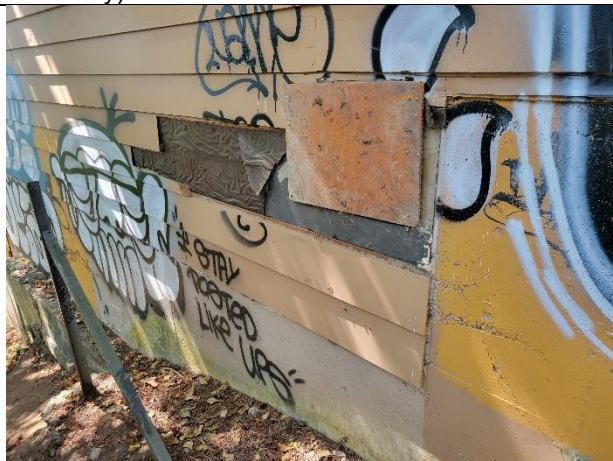
Damaged siding east elevation
