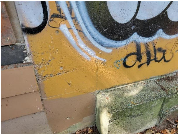
Some stem wall cracking – east elevation
