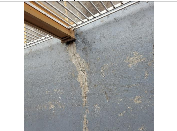
2 nd level concrete crack – trip hazard
