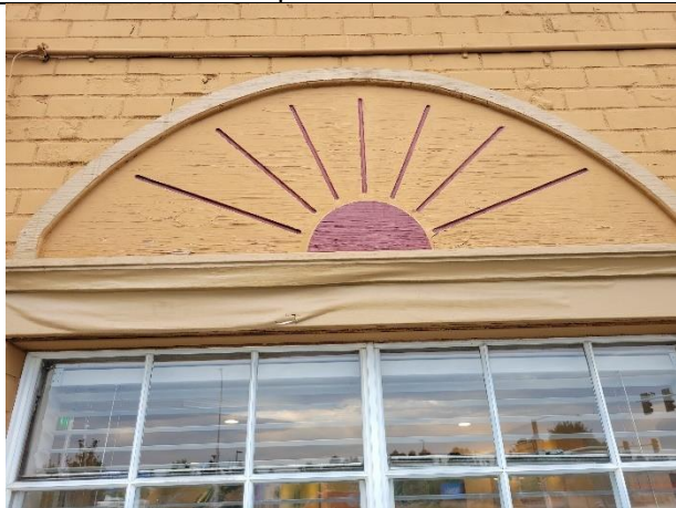
Wooden architectural feature – paint chipping
