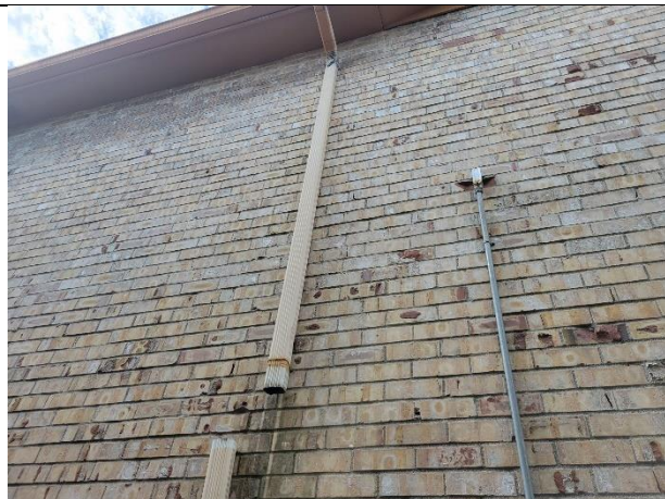
Disconnected downspout
