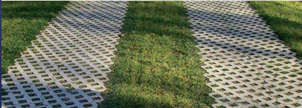
Permeable interlocking pavers
