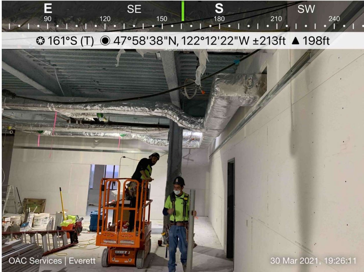
Similar view of Courtroom 4A in late March.
