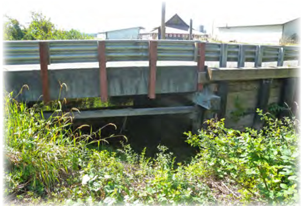
Portage Creek Bridge 311 on 43rd Ave NE in Arlington is a short span built in 1972. It's an example of one of our bridges that is a combination of wood and concrete construction.
