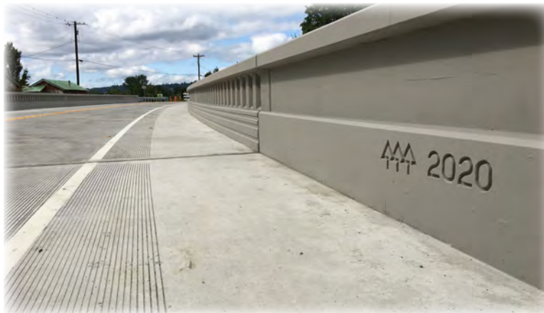
Riley Slough Bridge 155, a 12-span timber trestle with a concrete deck built in 1930, was replaced with a new three-span concrete bridge that was completed and opened in the summer of 2020. It is located on Tualco Road across Riley Slough southwest of Monroe.
