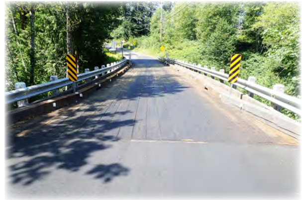
Jordan Creek Bridge 214.
