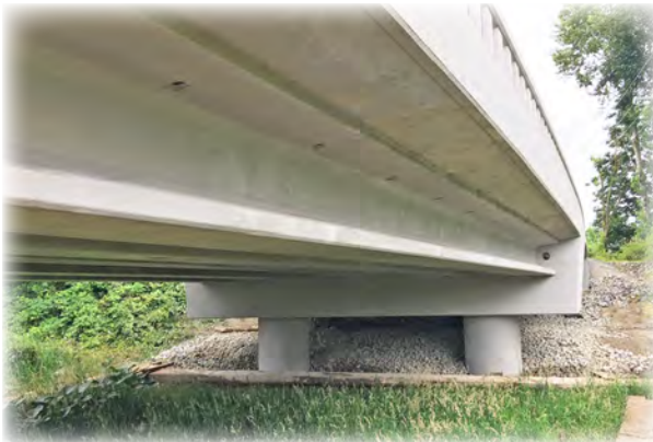
Riley Slough Bridge 155.
