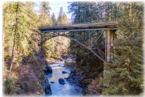
Granite Falls Bridge 102.
