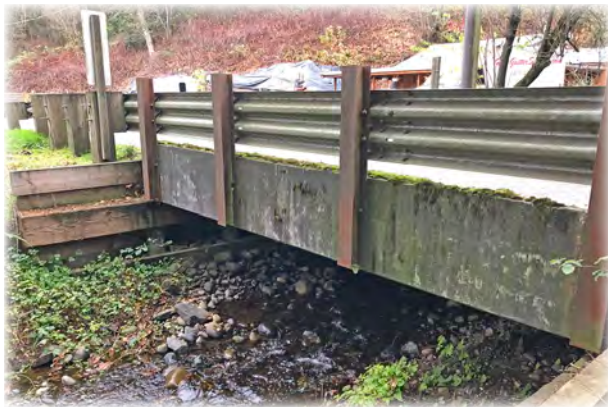
Richardson Creek Bridge 300.
