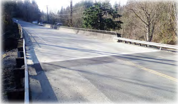
New slab at the east end of the bridge.
