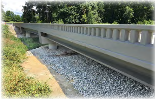
Riley Slough Bridge 155.
