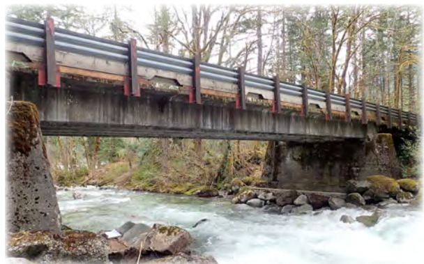
Trout Creek Bridge 494.
