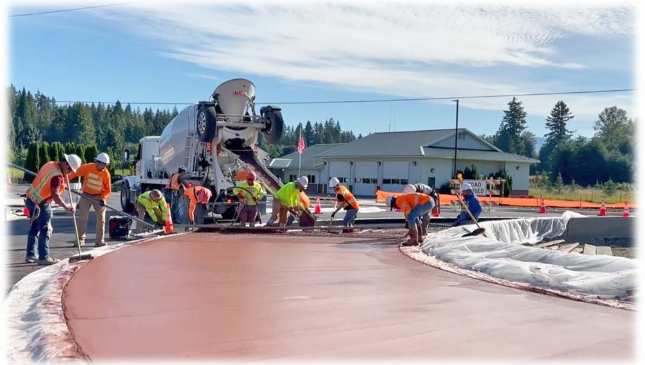
A roundabout is currently under construction at the 84 th St NE and 163 rd Ave NE intersection.
