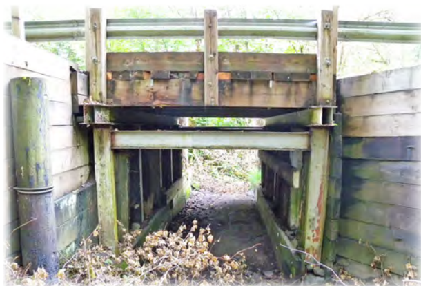
Everett Creek Bridge 565 located 3.5 miles northeast of Darrington on Crawford Loop Road was built in 1985. It is a short span with an overall length of 15 feet (NBIS length of 12 feet) and has a fish passage restriction. The bridge is planned to be replaced with a longer structure.
