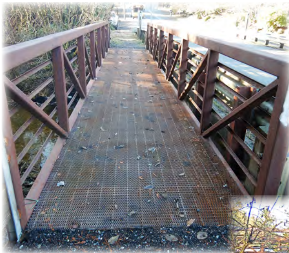
The recycled pre-fabricated steel pedestrian bridge is a major improvement for pedestrians using Swamp Creek Bridge 459.
