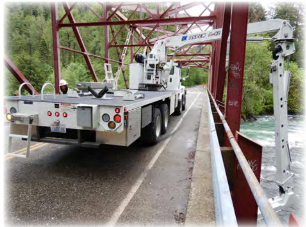
Red Bridge 538 on the Mountain Loop Highway. County and WSDOT inspectors are inspecting the bridge's steel truss via a WSDOT UBIT.
