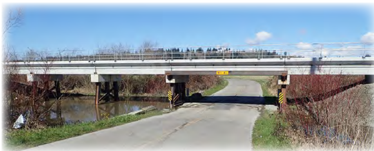
Olsen Road Railroad Underpass is height restricted. In 2019 BNSF replaced an all timber trestle with a steel and concrete bridge.
