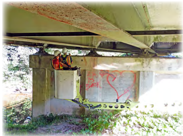
Pilchuck Creek Bridge 626, built in 1933, requires a Special Feature Inspection of the steel pins every 72 months. Ultrasonic Testing (UT) equipment provides an effective, non-destructive method to assess the condition of steel members.
