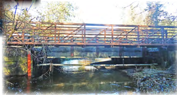
The recycled pre-fabricated steel pedestrian bridge is a major improvement for pedestrians using Swamp Creek Bridge 459.
