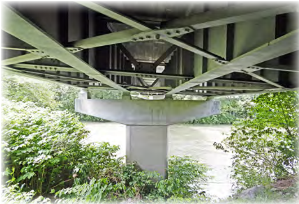
Larson Bridge 101 is a three span bridge built in 1962 prior to current seismic design standards. The bridge carries Larson Rd over the South Slough of the Stillaguamish River in Silvana. Snohomish County is seeking federal funds to support a seismic retrofit project that would reduce vulnerability to collapse in a heavy seismic event.
