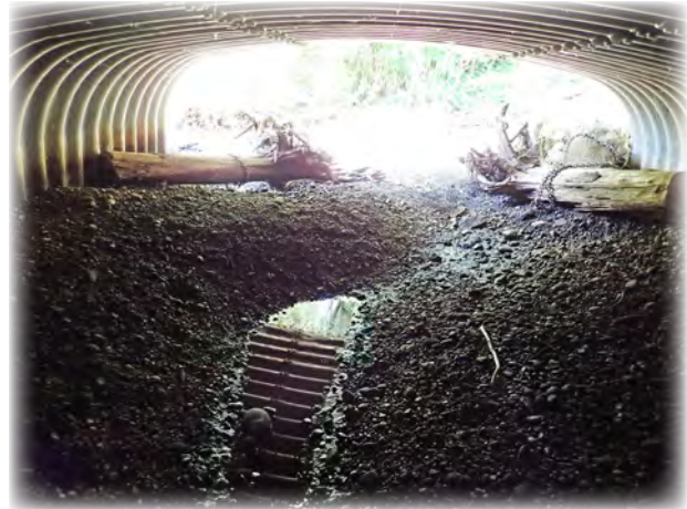
Bridge 14 is a corrugated aluminum culvert carrying Swamp Creek at the intersection of Gibson Road and Admiralty Way. A scour mitigation work order was completed in the fall of 2017.
