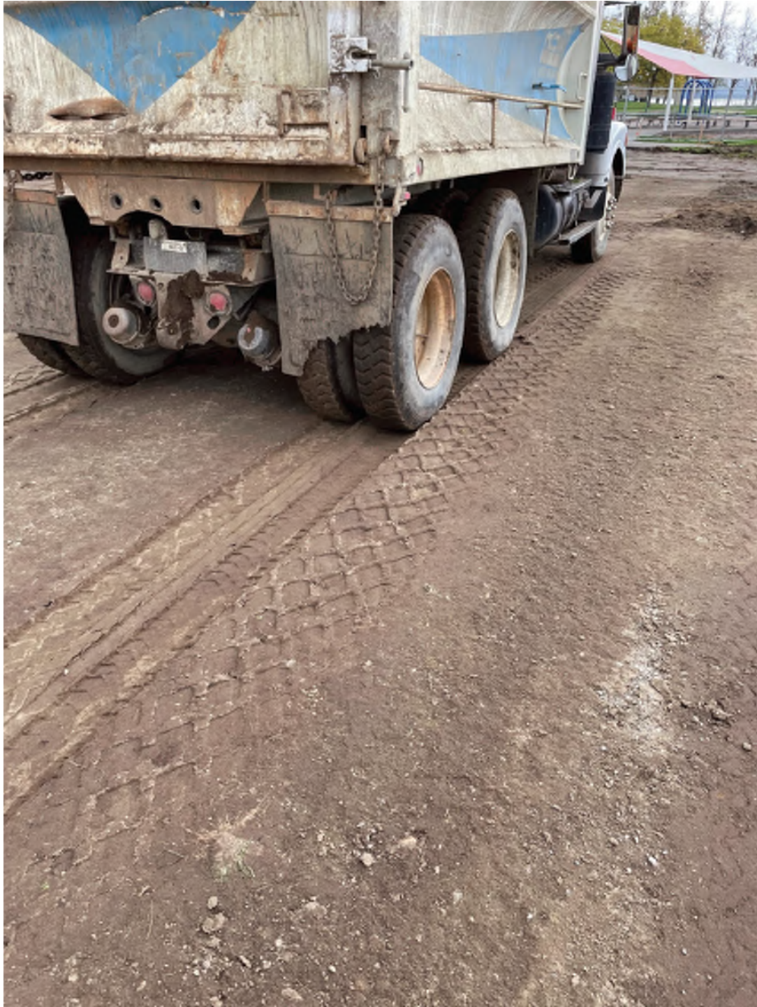
Photograph 2 – Proof Rolling of Subgrade
