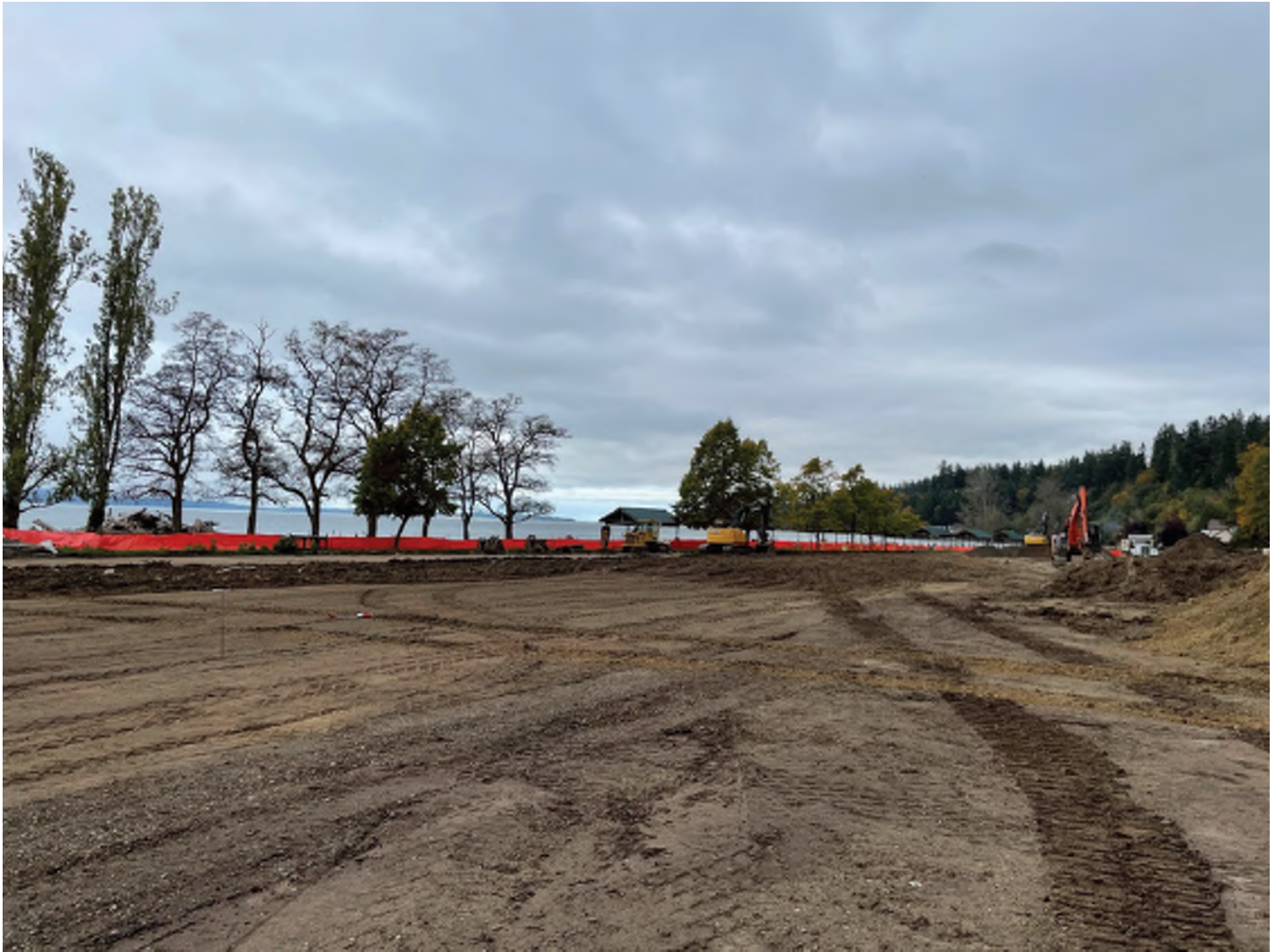
Photograph 1 – Proposed Parking Lot Subgrade
