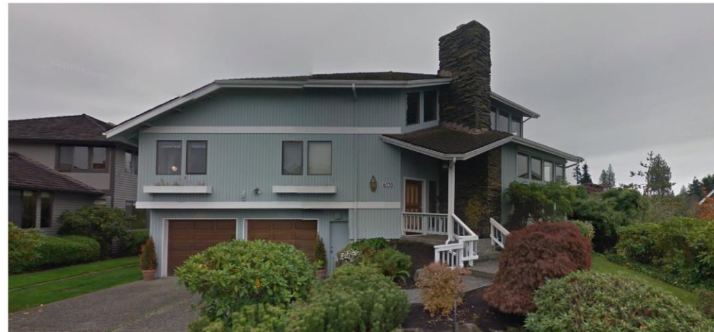
Existing 3-Story House in a 1970s-era PRD (Picnic Point)
