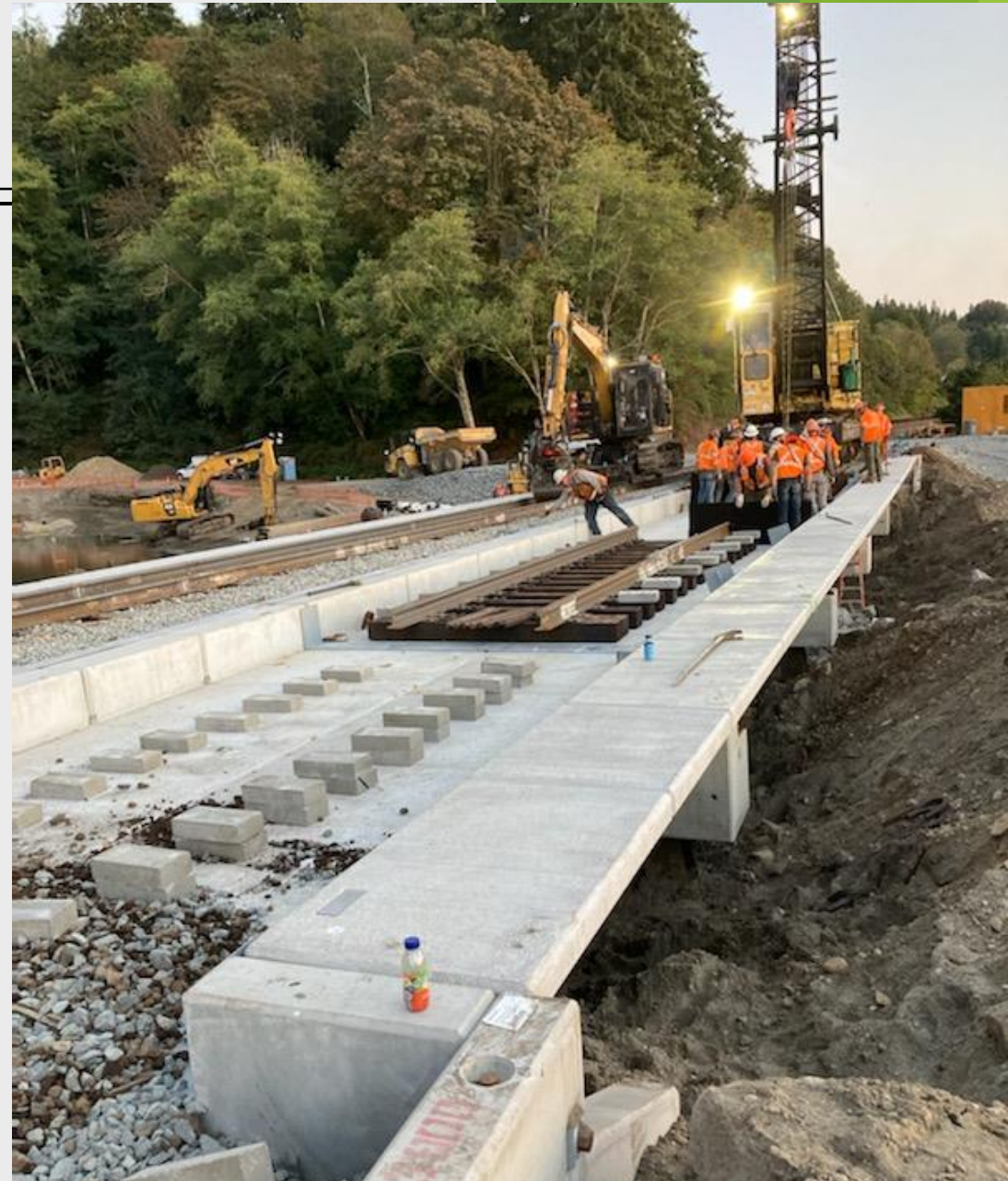
Meadowdale Bridge Install
