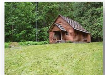
The project will encompass the completion of the roof replacement for the Suiattle Guard Station. This building is listed on the National Register of Historic Places (NRHP). Roof replacement with hand-split cedar shingles is planned to maintain the historic integrity of the building.
