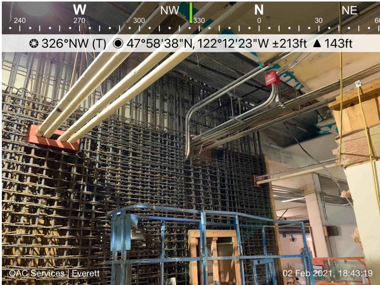
Rebar cage for basement segment of shearwall in early February.
