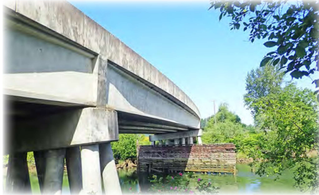
Ebey Slough Bridge 3 built in 1976 on Home Acres Road is one of the county's Lifeline Route bridges. It is located in Everett in the Snohomish River valley 1.3 miles east of Lowell and the Snohomish River.
