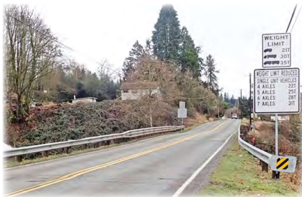
Cattle Pass Bridge 183 on Lowell-Larimer Road has new weight limits posted.
