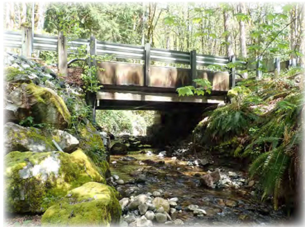
Hogarty Creek Bridge 636 on Reiter Rd in Sultan is a short span built in 1997. It’s an example of one of our bridges that is a combination of wood and concrete construction.
