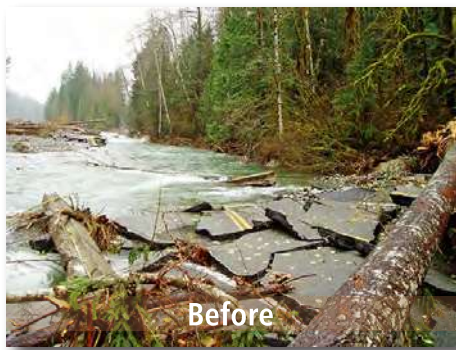
Looking upstream at the flood damaged Index-Galena Road near mile 6.9 in 2006.
